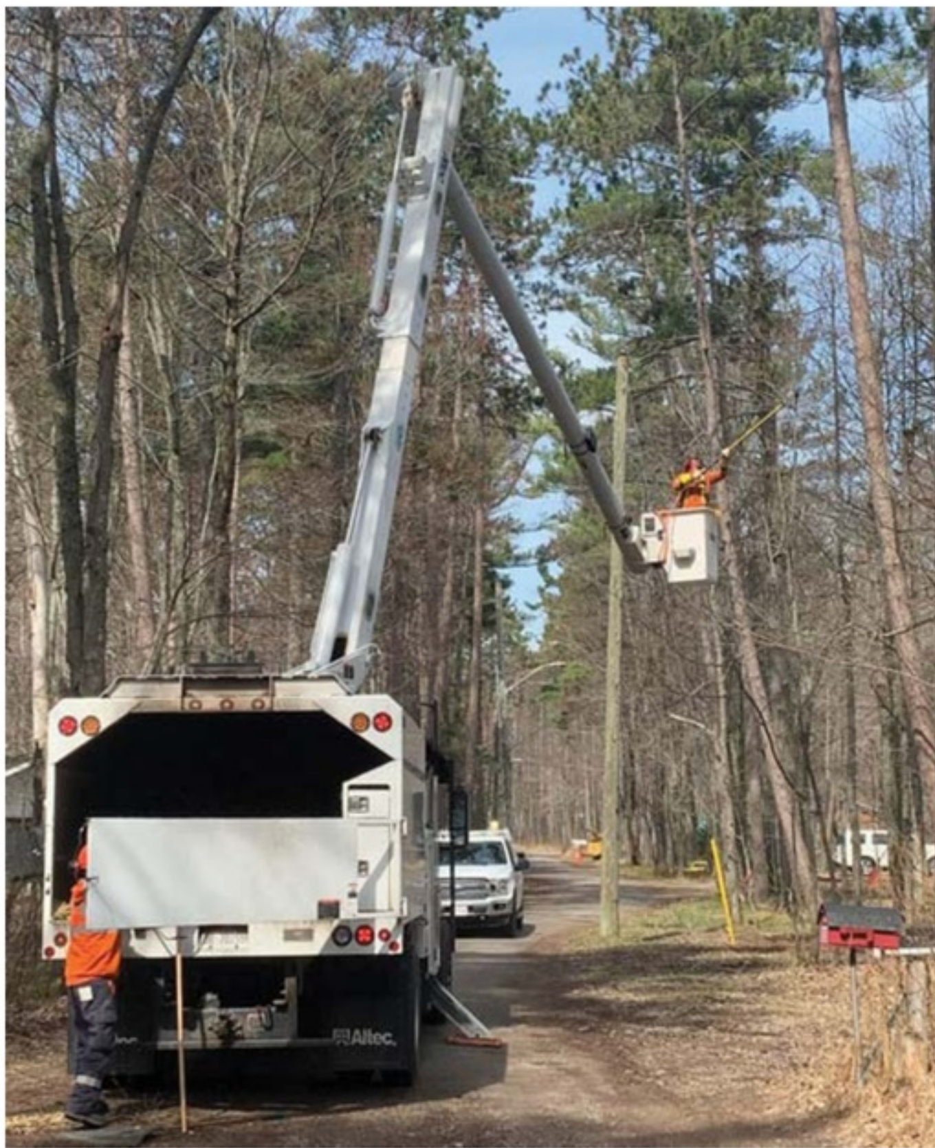
Brad Gibbs, journeyman utility arborist, clears lower limbs that are within proximity to the line. He is using rubber gloves and dielectric hydraulic pruners to get a safe clearance to best perform the rest of the trim.
